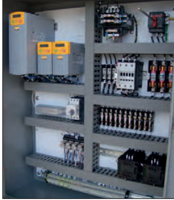
3 Drive System with Temperature Control
