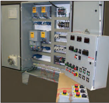
Completed System Test
